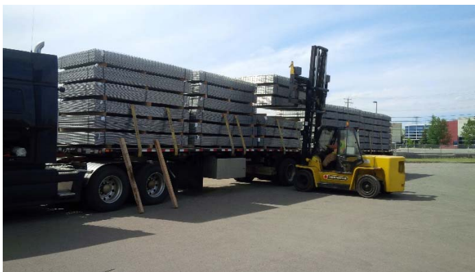
Loading a truck of welded wire reinforcement
