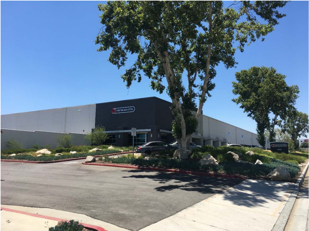
San Bernardino Facility
