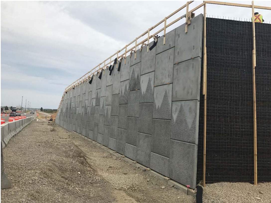
Application of mesh for earth reinforcement of highways and roadways.
